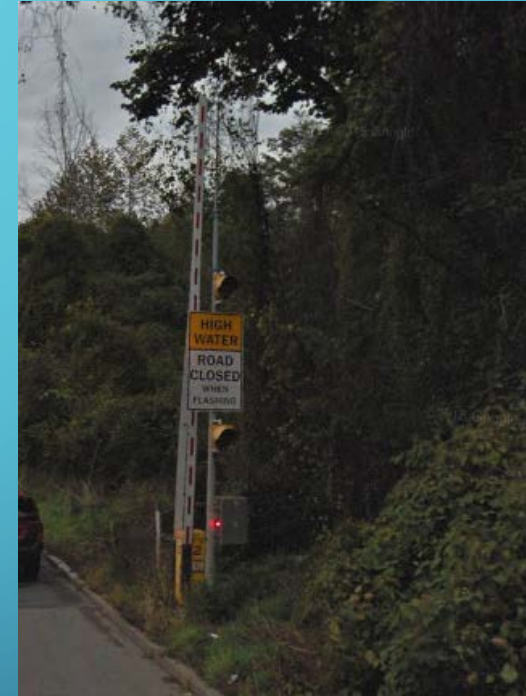
Flood Warning System
