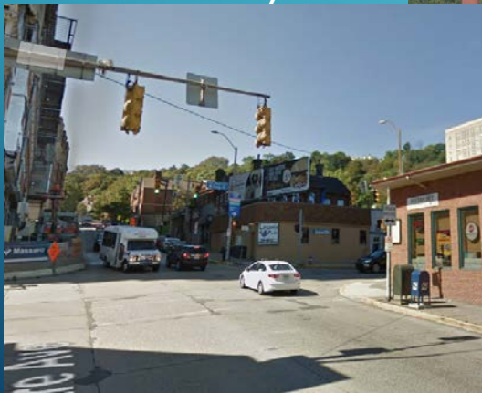
Adaptive Signal Control
